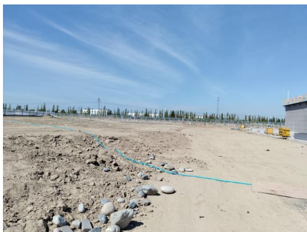
拟建变电站西侧
